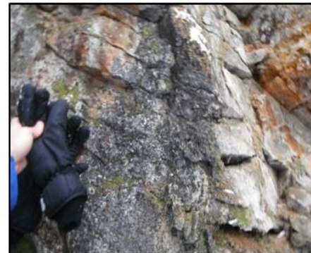
Figure 2 & 3: area at south-west wall of the mine pit. View toward south.
